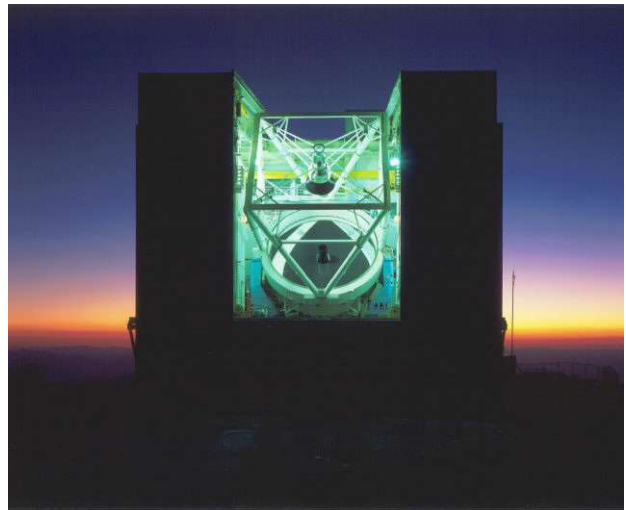
Fig. 1. The Converted MMT at sunset. Photo by H. Lester.
