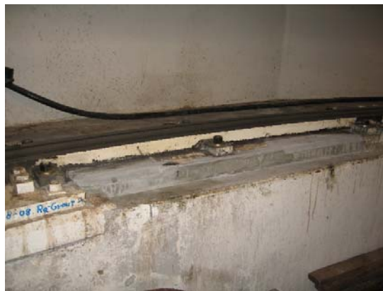
Grout is successfully placed; curing cycle is underway.
